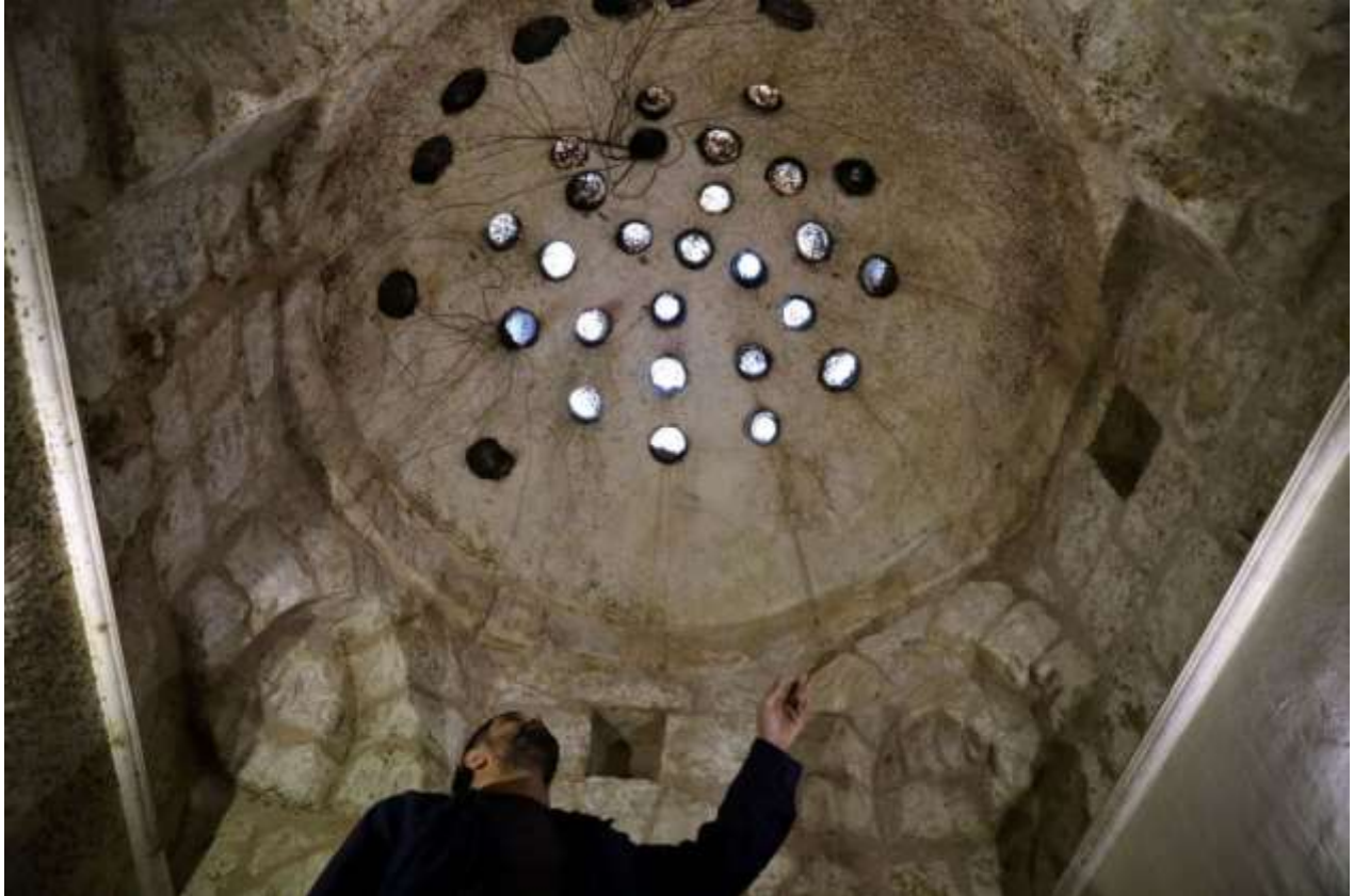
Palestinian worker Ibrahim Al Hawamdeh points at the ceiling of the first traditional Turkish bath (Hamam) in the West Bank city of Hebron, November 29, 2021. PHOTO: EPA-EFE
